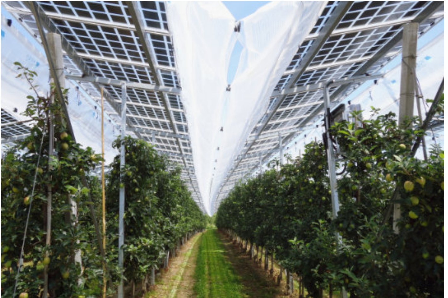
Agriphotovoltaik in Kressbronn
